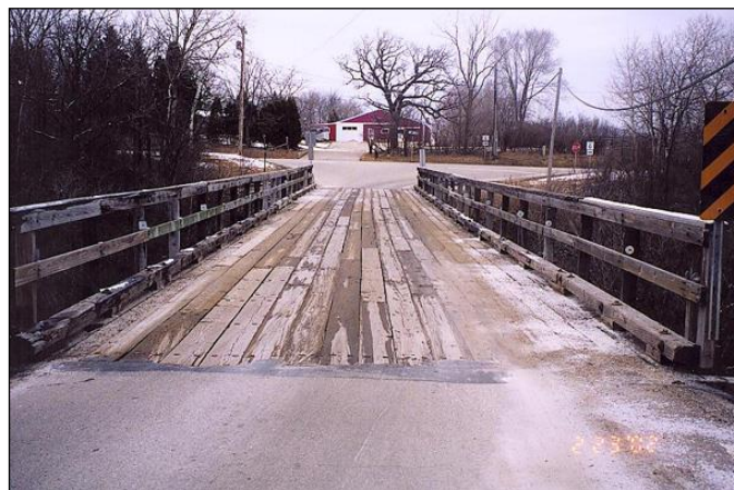
Figure 2.3.5-1: Timber Plank Deck (Top Surface Evaluated as Wearing Surface – Bare).
