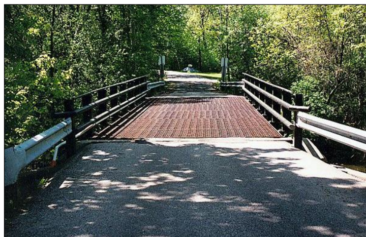
Figure 2.3.4.1-1: Open Grid Steel Deck.
