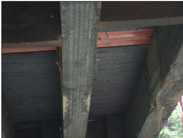
Figure 2.3.5.1-1: Timber Deck – Condition State 1.
