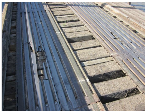
Figure 2.3.5-2: Steel Running Boards on a Timber Deck.
