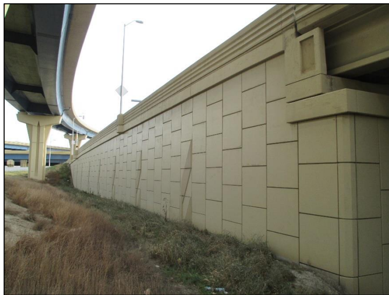
Figure 4.4.1-1: MSE “Fill” Wall
