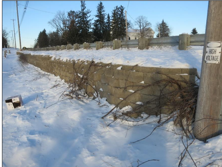
Figure 4.4.4-5: Segmented Modular Block Gravity Wall.
