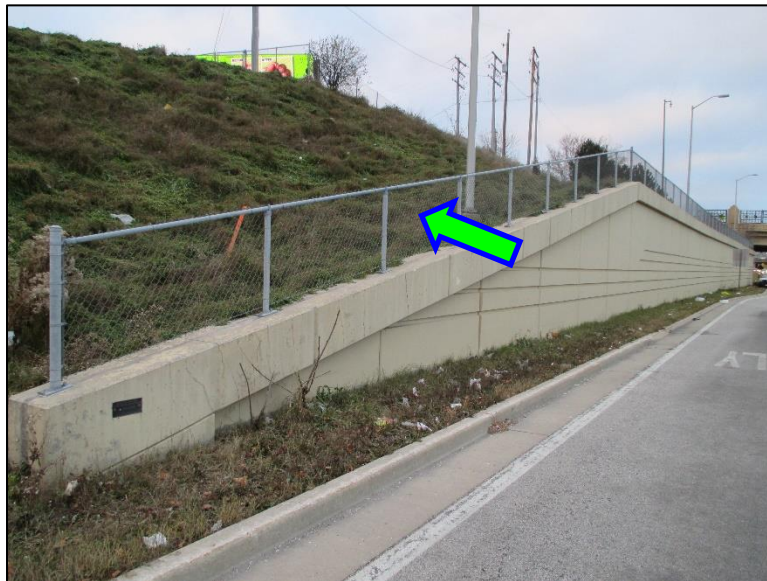
Figure 4.4.5-8: Protective Screening Fastened to a Horizontal Coping. Note the Screening is Not Adjacent to a Sidewalk.
