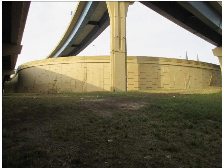
Figure 4.4.4-8: MSE Precast Concrete Panel Facing Wall.
