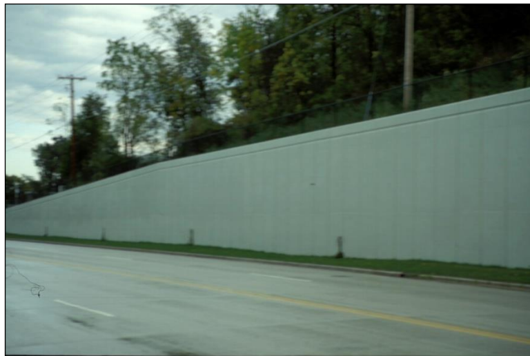
Figure 4.4.4-1: Cast-in-Place Concrete Cantilever Wall.
