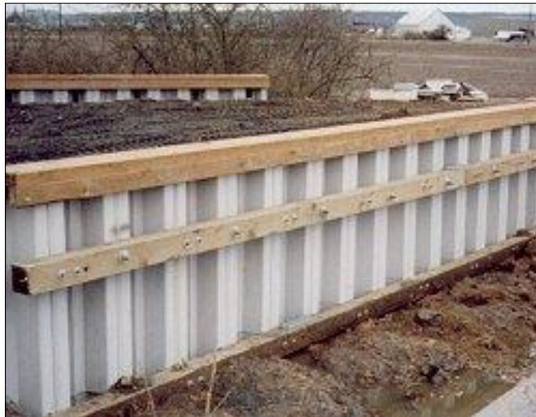
Figure 4.4.4-17: Vinyl Sheet Piling Retaining Wall.
