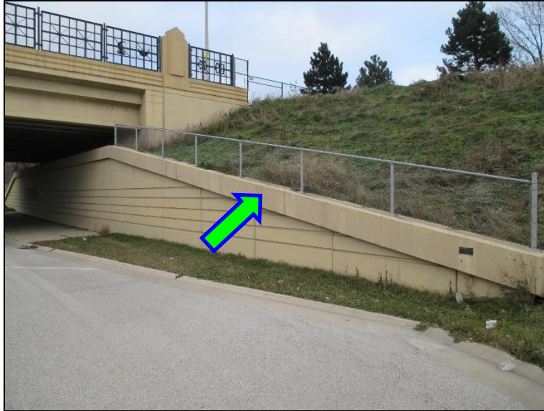
Figure 4.4.5-10: Cast-In-Place Horizontal Coping
