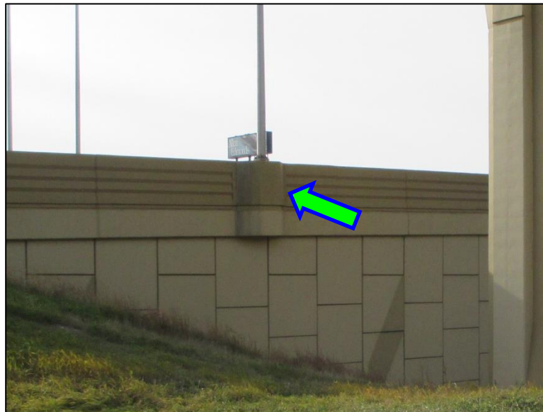
Figure 4.4.5-7: Luminaire Base Placed in Coping and Barrier Wall.
