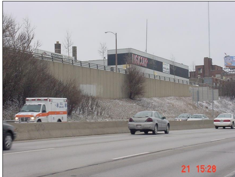
Figure 4.4.4-2: Cast-in-Place Concrete Cantilever Wall.
