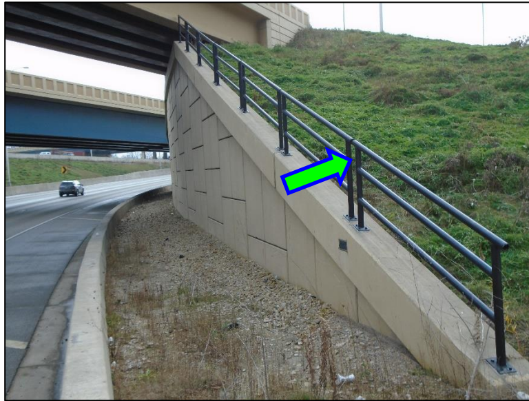
Figure 4.4.5-5: Decorative Rail atop a Horizontal Coping.
