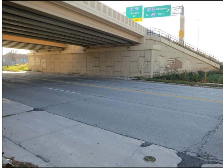
Figure 4.4.5-3: Aesthetic Treatment Form-Lined Precast Concrete Panels.
