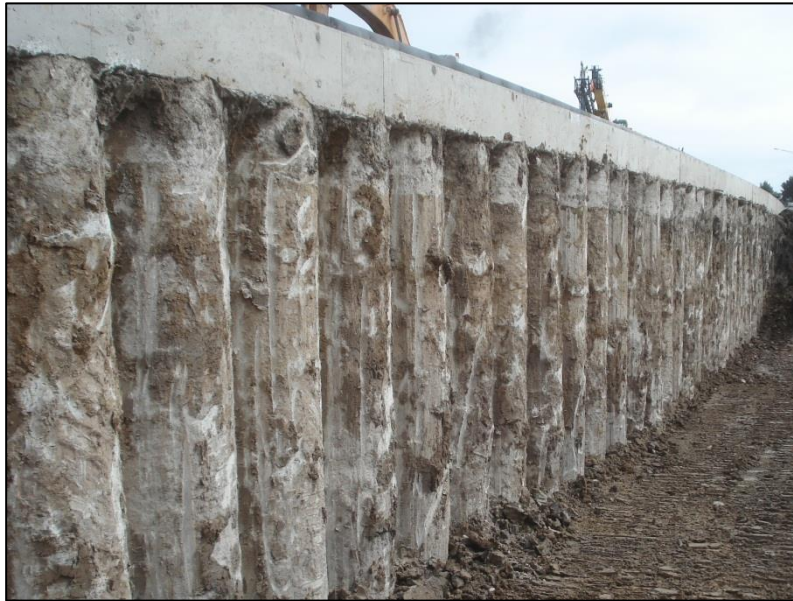
Figure 4.4.4-15: Secant Wall Constructed as Tunnel Wall.
