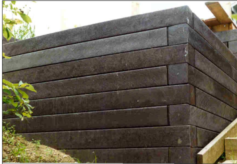
Figure 4.4.2-24: Plastic Lumber Retaining Wall.
