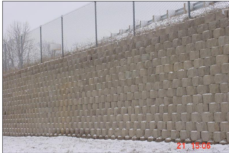
Figure 4.4.4-7: Segmented Modular Block MSE Wall.
