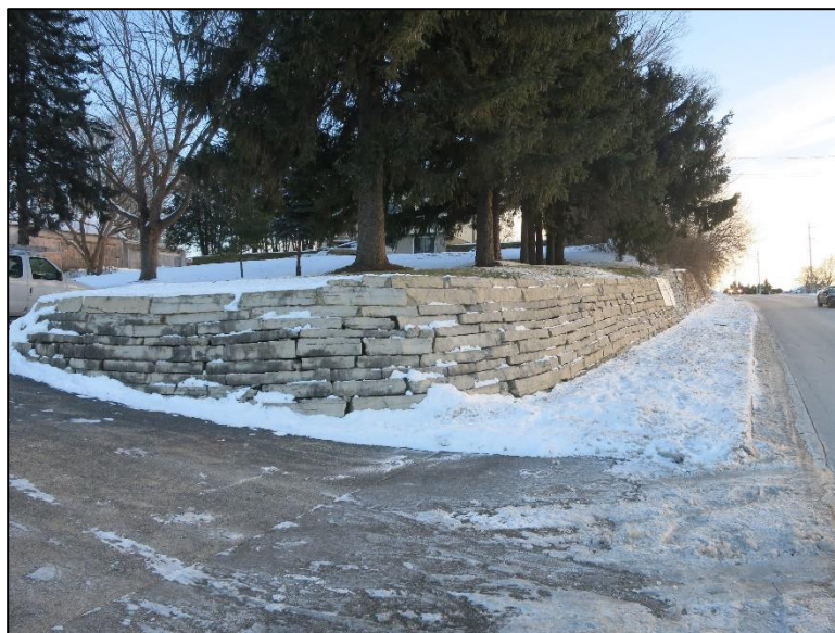
Figure 4.4.4-6: Lannon Stone (Limestone) Block Gravity Wall.
