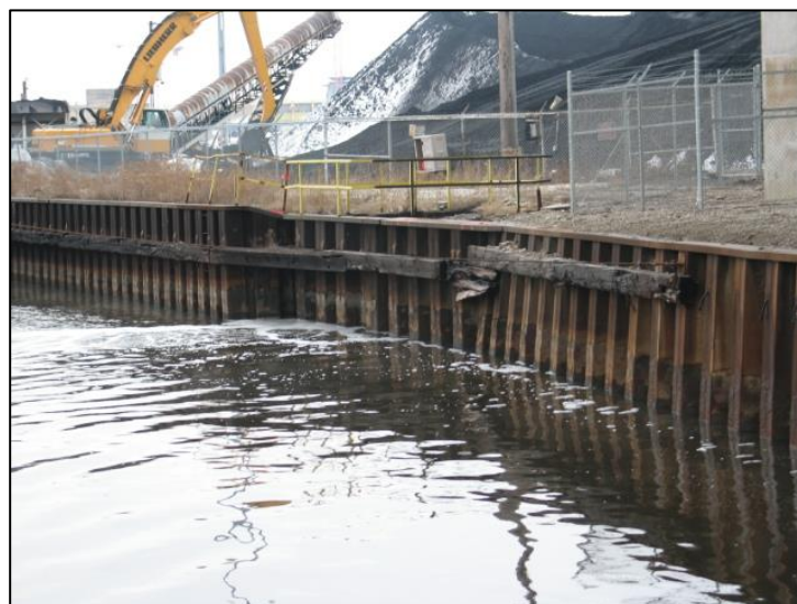
Figure 4.4.1-3: Steel Sheetpile Dockwall
