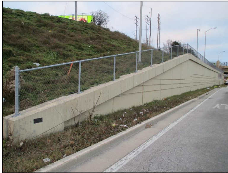
Figure 4.4.1-2: CIP “Cut” Wall
