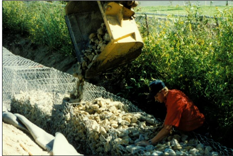
Figure 4.4.4-3: Gabion Gravity Crib Wall Under Construction.
