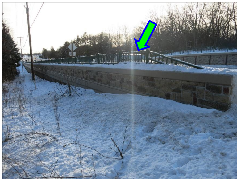
Figure 4.4.5-6: Decorative Rail atop a Bridge Rail Element.
