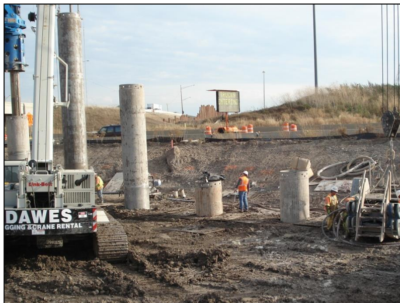
Figure 4.4.4-14: Secant Wall Construction.
