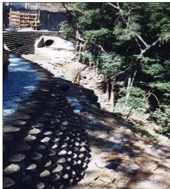
Figure 4.4.2-25: Geotextile Grid Cell Retaining Wall.
