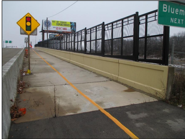
Figure 4.4.5-11: Concrete Sidewalk Along Top of Retaining Wall.
