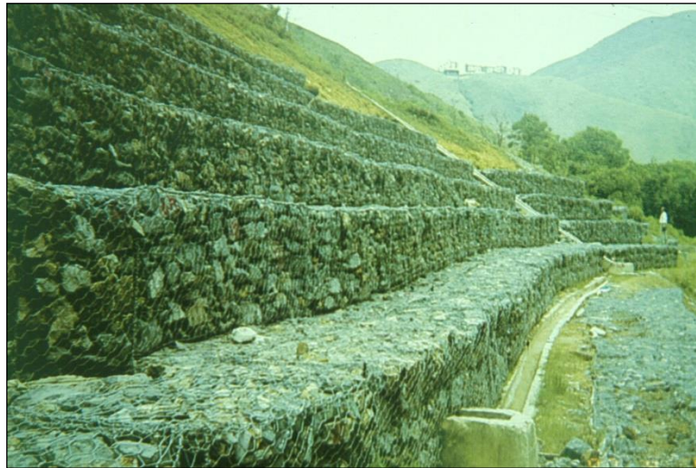
Figure 4.4.4-4: Tiered Gabion Gravity Crib Wall.
