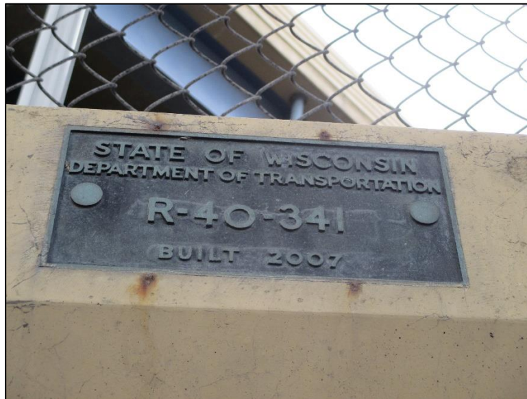
Figure 4.4.5-4: Retaining Wall Name ID Plaque.
