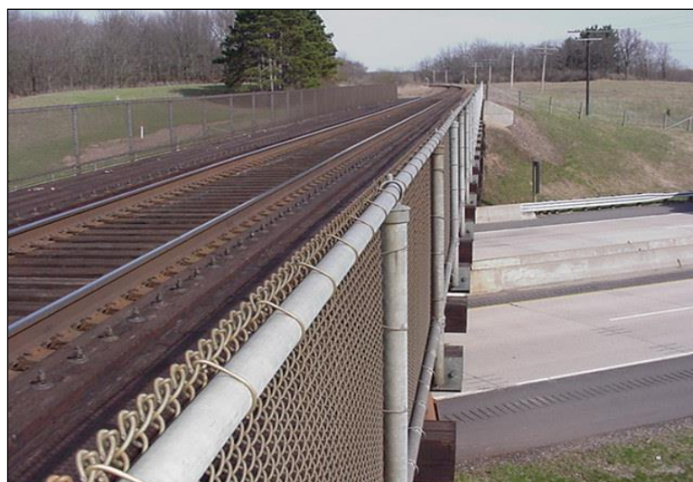
Figure 4.8.2-1: Railroad Bridge Top View.
