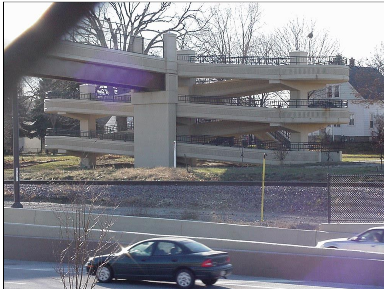
Figure 4.8.3-2: Pedestrian Bridge Entrance/Exit Ramp.
