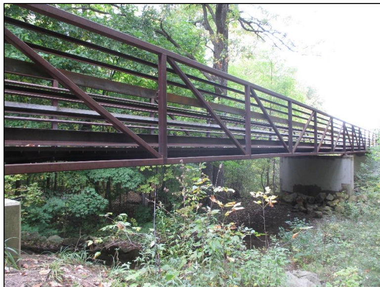
Figure 4.8.3-4: Steel Thru Truss Pedestrian Bridge.
