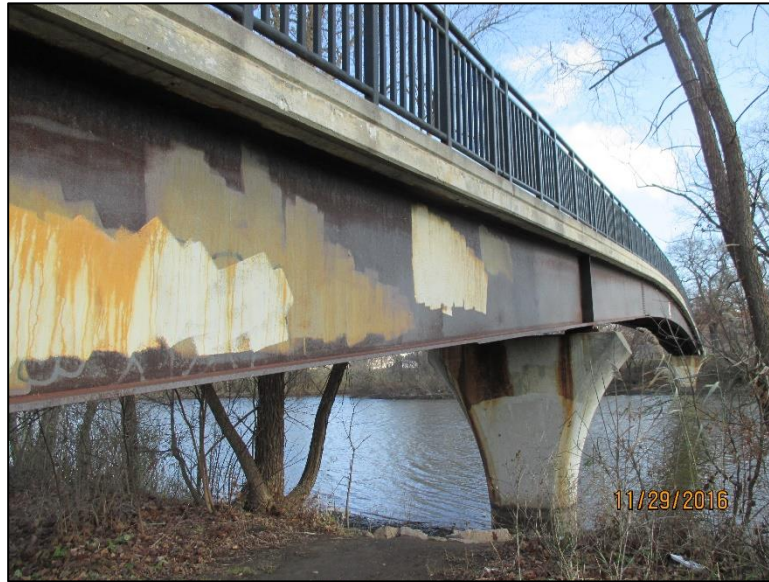
Figure 4.8.3-3: Non-Redundant Steel Girder Pedestrian Bridge.
