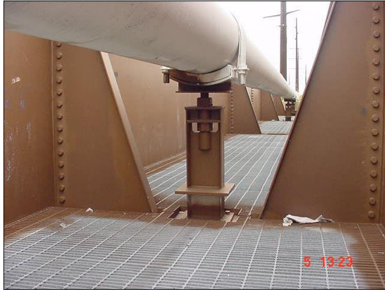
Figure 4.8.4-2: Pipeline to Bridge Connection.
