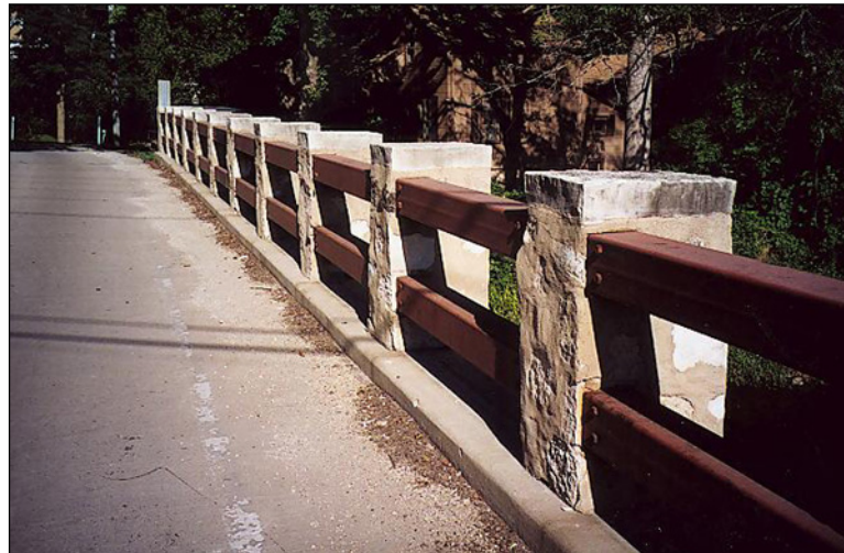
Figure 2.6.7.1-1 Metal Railing with Masonry Posts – Condition State 1
