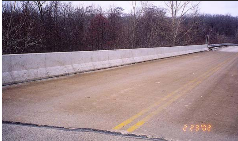
Figure 2.6.7.2-1 Concrete Bridge Railing - Condition State 1
