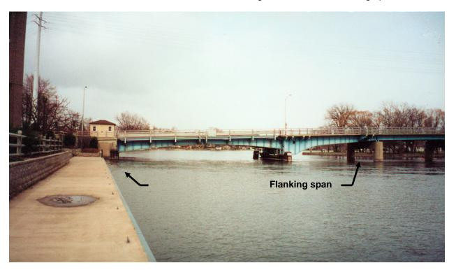
**Figure 3.2.3-3:** Double-Leaf Rolling Lift Bascule, Racine Street Bridge in Menasha. Note: Left leaf rolls on a bascule abutment, right leaf rolls on a flanking span.
