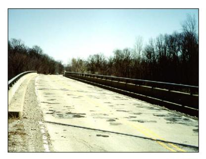
Figure 5.11.1-1: Bridge Deck with Asphalt Overlay and Extensive Patching.
