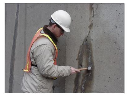
Figure 5.3.1-1: Inspector Hammer Sounding a Bridge Abutment.
