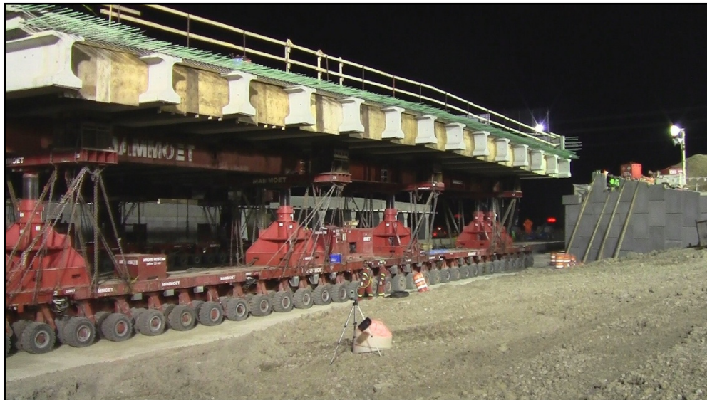
Figure 7.1-7 Self Propelled Modular Transporters Moving a Bridge
