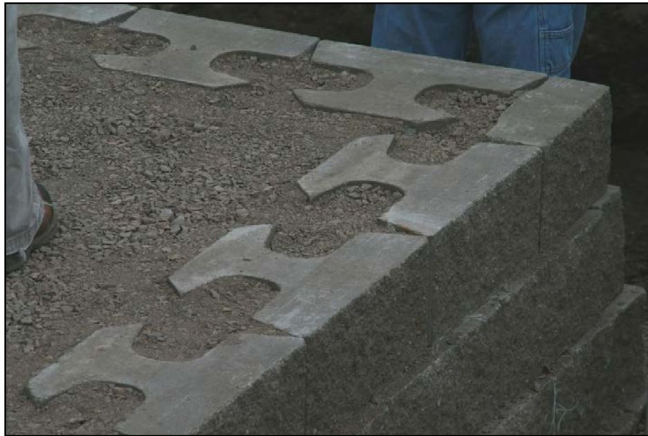
Figure 7.1-5 GRS Abutment Layer During Construction
