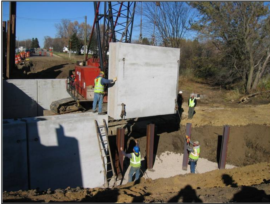
Figure 7.1-2 Prefabricated Abutment
