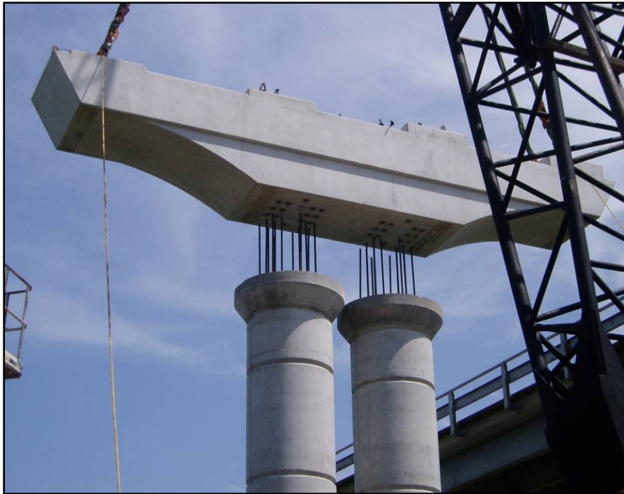
Figure 7.1-1 Prefabricated Pier Cap
