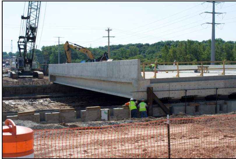
Figure 7.1-6 Lateral Sliding
