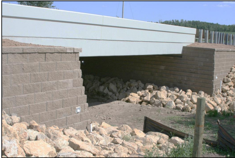
Figure 7.1-4 GRS-IBS Structure
