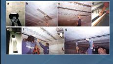
C. Locate Strips/Check Surface D. Clean and Prepare FRP Strips G. Roll Out to Ensure Total Contact
