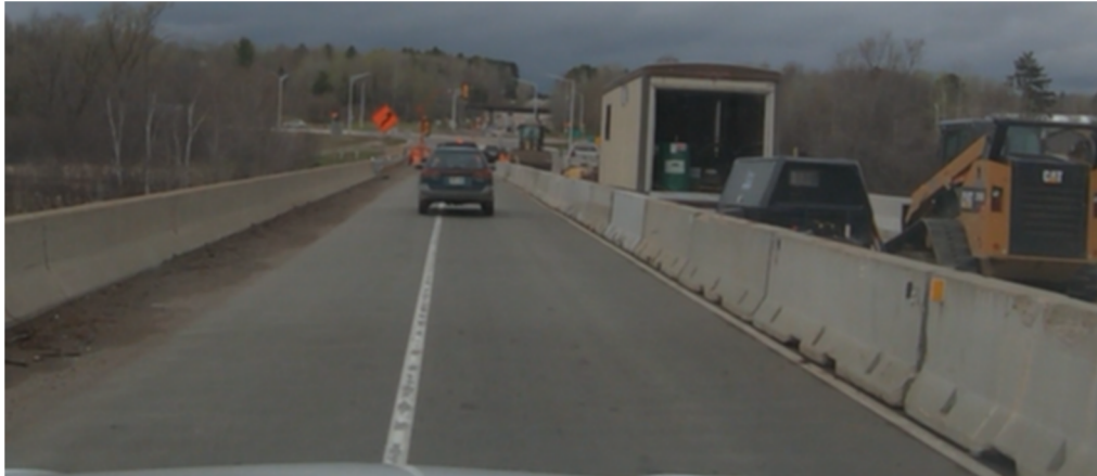
Figure 11: Missing Pavement Markings (End Lines and Skips)
