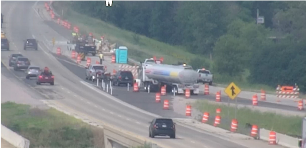
Figure 6: Off-Ramp without Proper Deceleration Length
