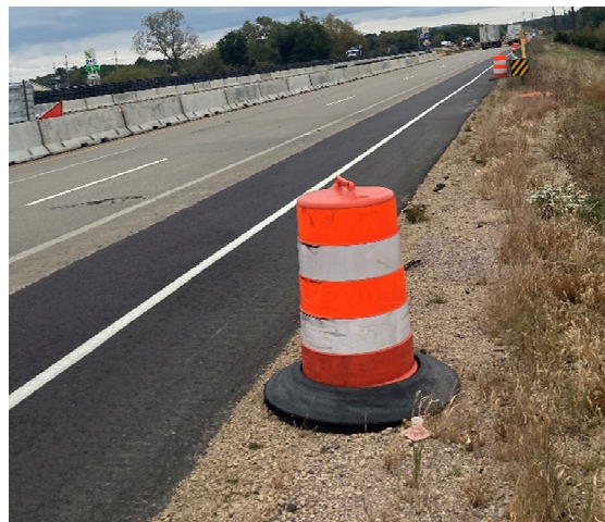
Figure 9: Temporary Pavement
