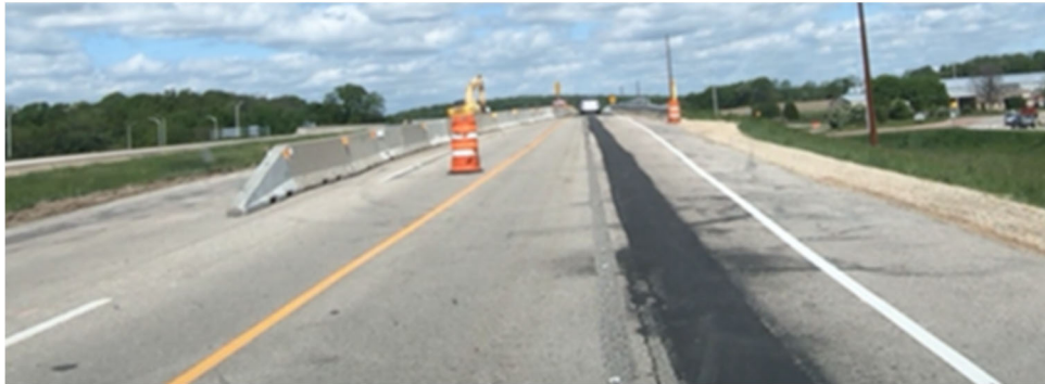
Figure 4: Contractor Access Point, Accessible Behind Barrier Wall
