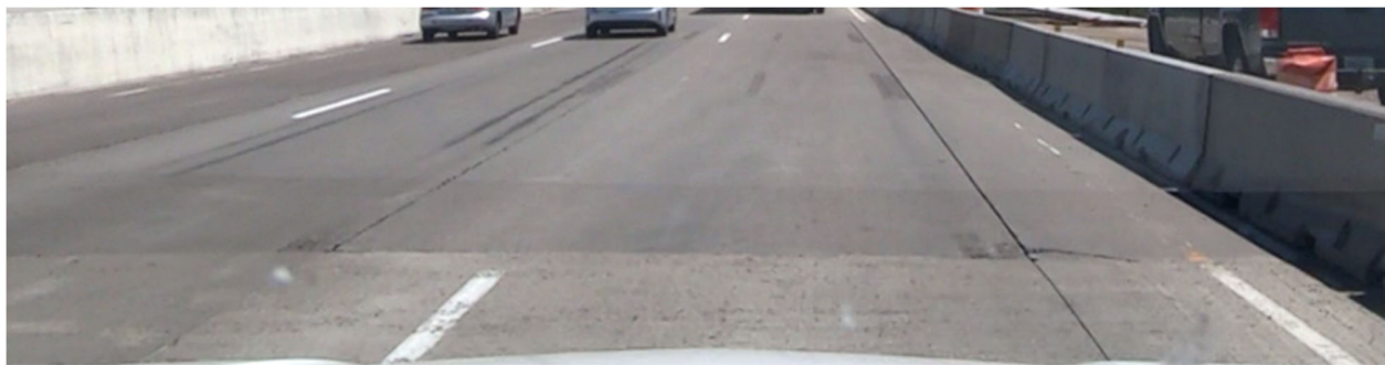
Figure 11: Missing Pavement Markings (End Lines and Skips)
