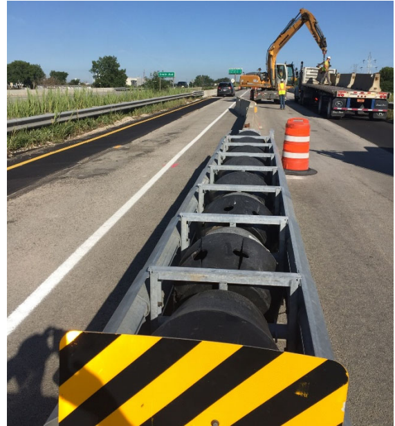
Figure 2: Crash Cushion at End of Barrier, Narrowed Work Zone at the Bridge
