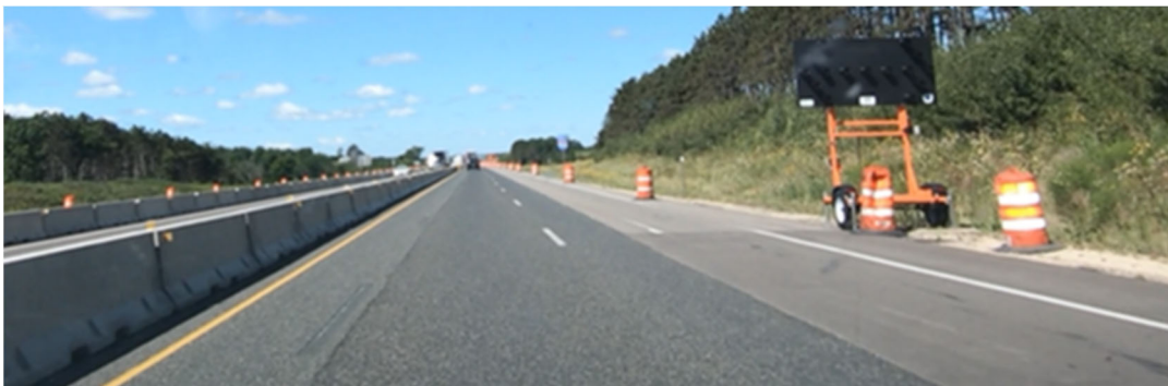
Figure 1: Bi-Directional Traffic Separated by Barrier Wall, Narrowed Lanes, Temporary Pavement
