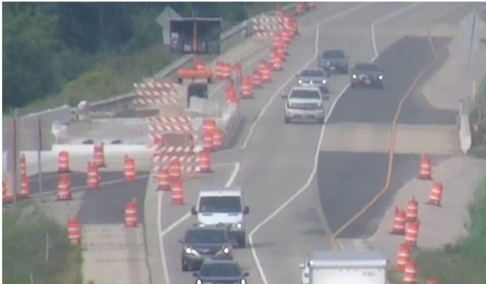
Figure 6: Off-Ramp without Proper Deceleration Length
