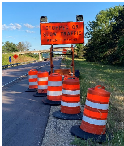
Figure 7: Basic Queue Warning System
