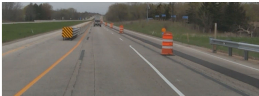
Figure 3: Crash Cushion at end of Barrier
