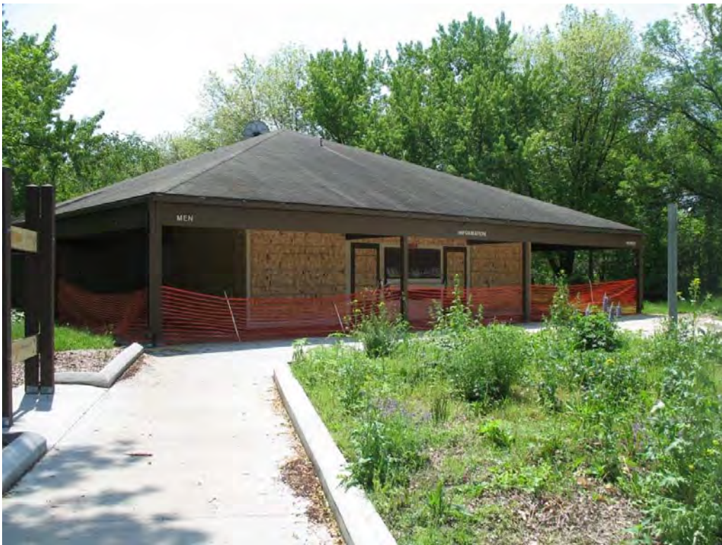
Main Rest Area Building
