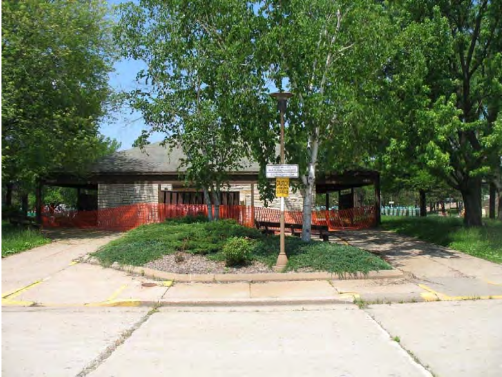
Main Rest Area Building
