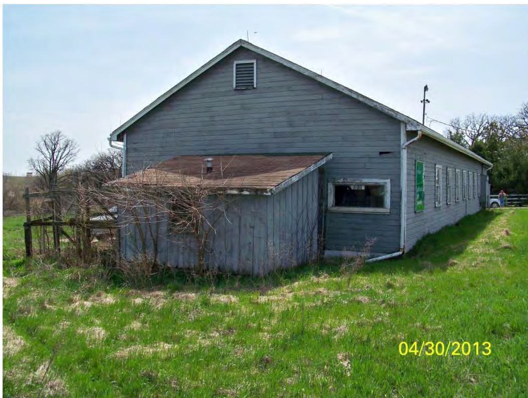
Machine/Storage Building with Coop (east side)
