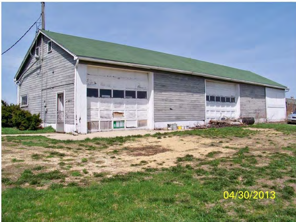
Machine/Storage Building (south side)
