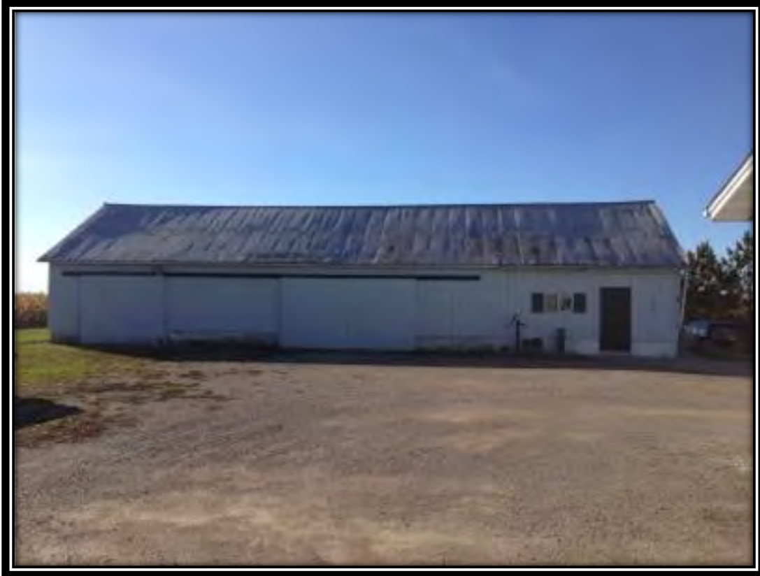
Front view of outbuilding
