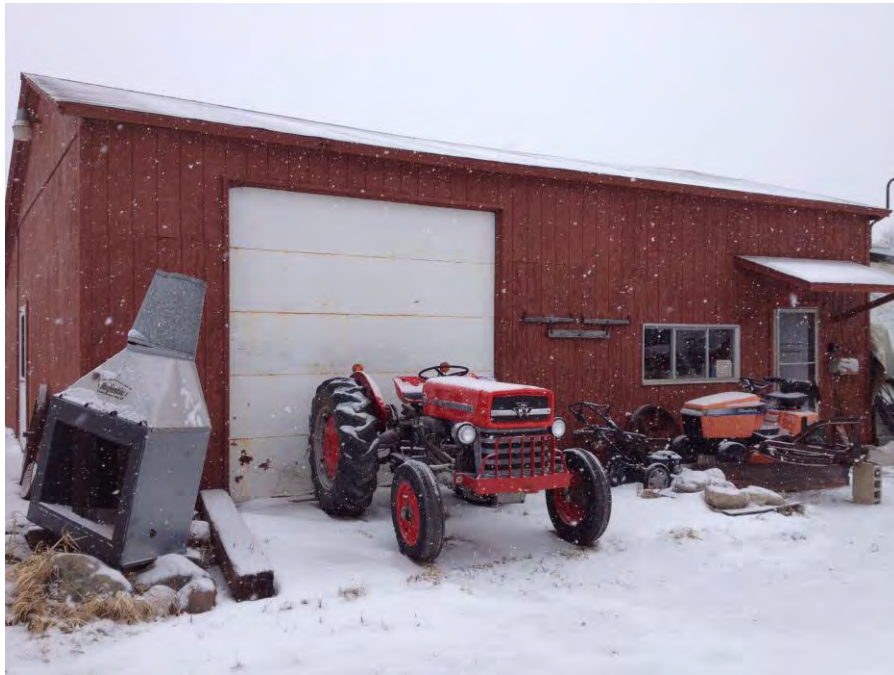
View of shop building in the fee taking area
