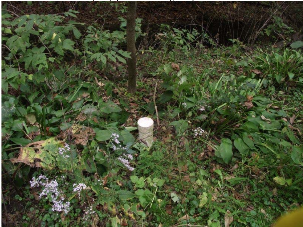
Possible septic pipe near drainage way south of house
