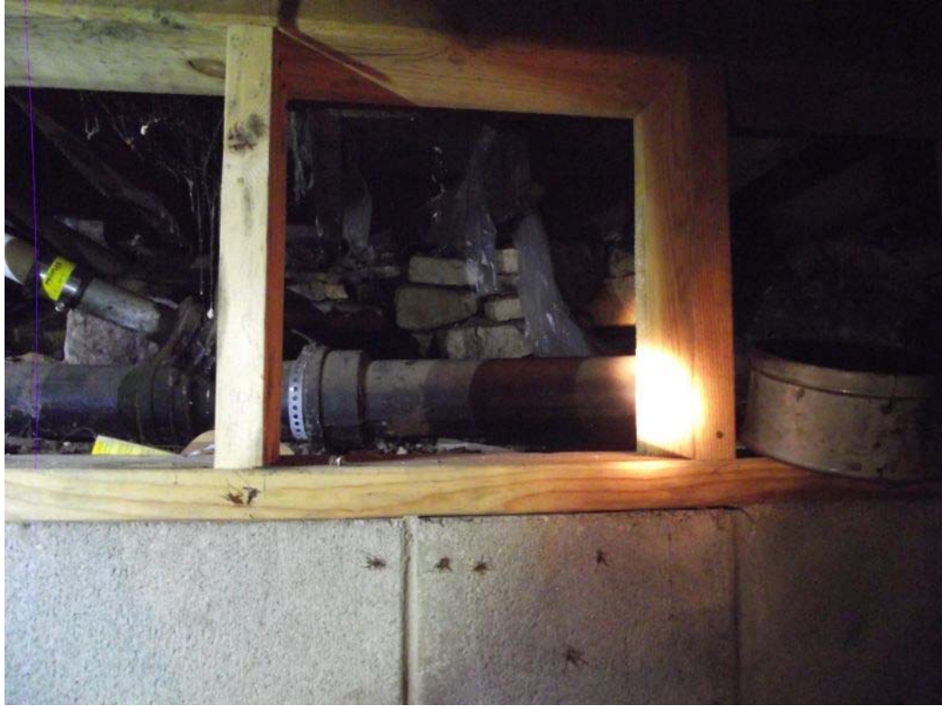
Septic pipes in crawl space under kitchen
