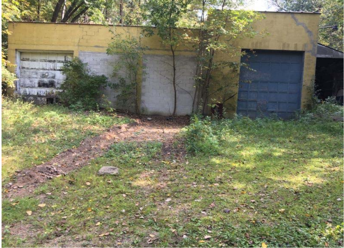
Front side of warehouse – facing east
