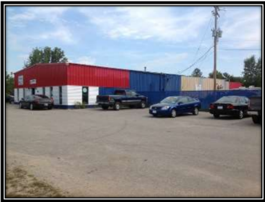
West and south (rear) walls of subject building looking northeast
