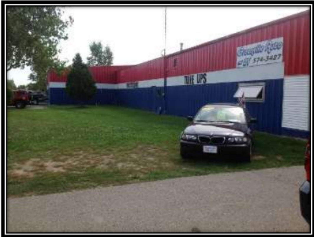
North (front) wall of subject building looking east
