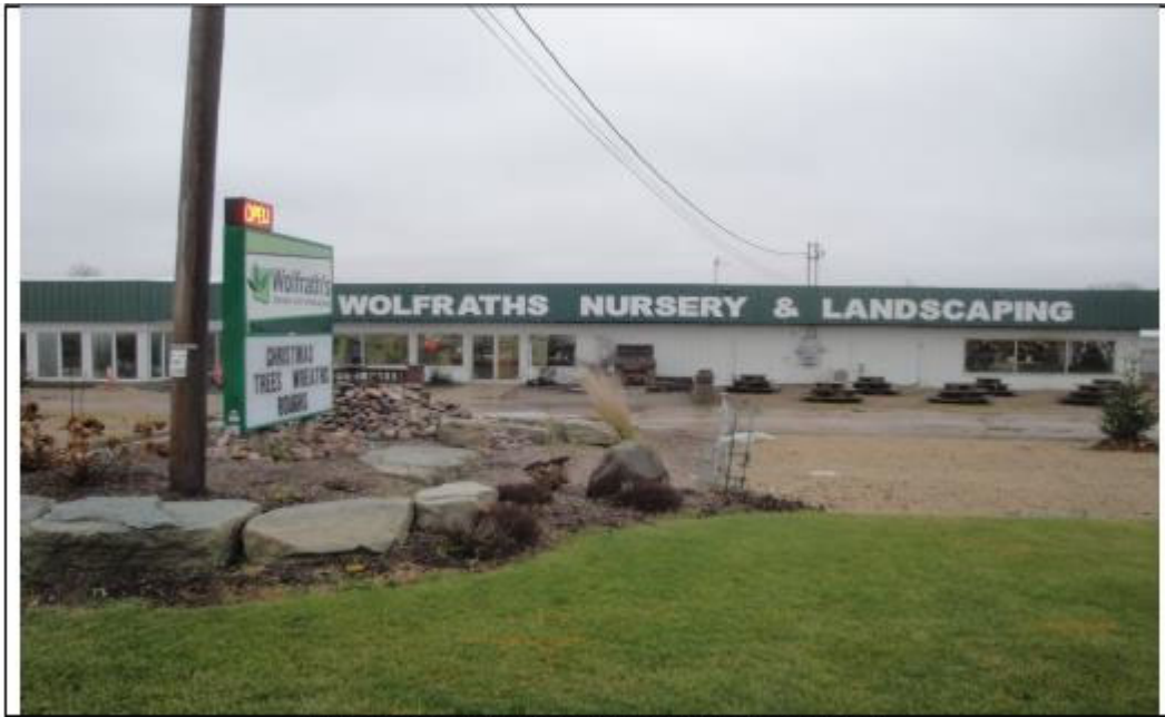
LOOKING NORTH AT THE SUBJECT SITE
