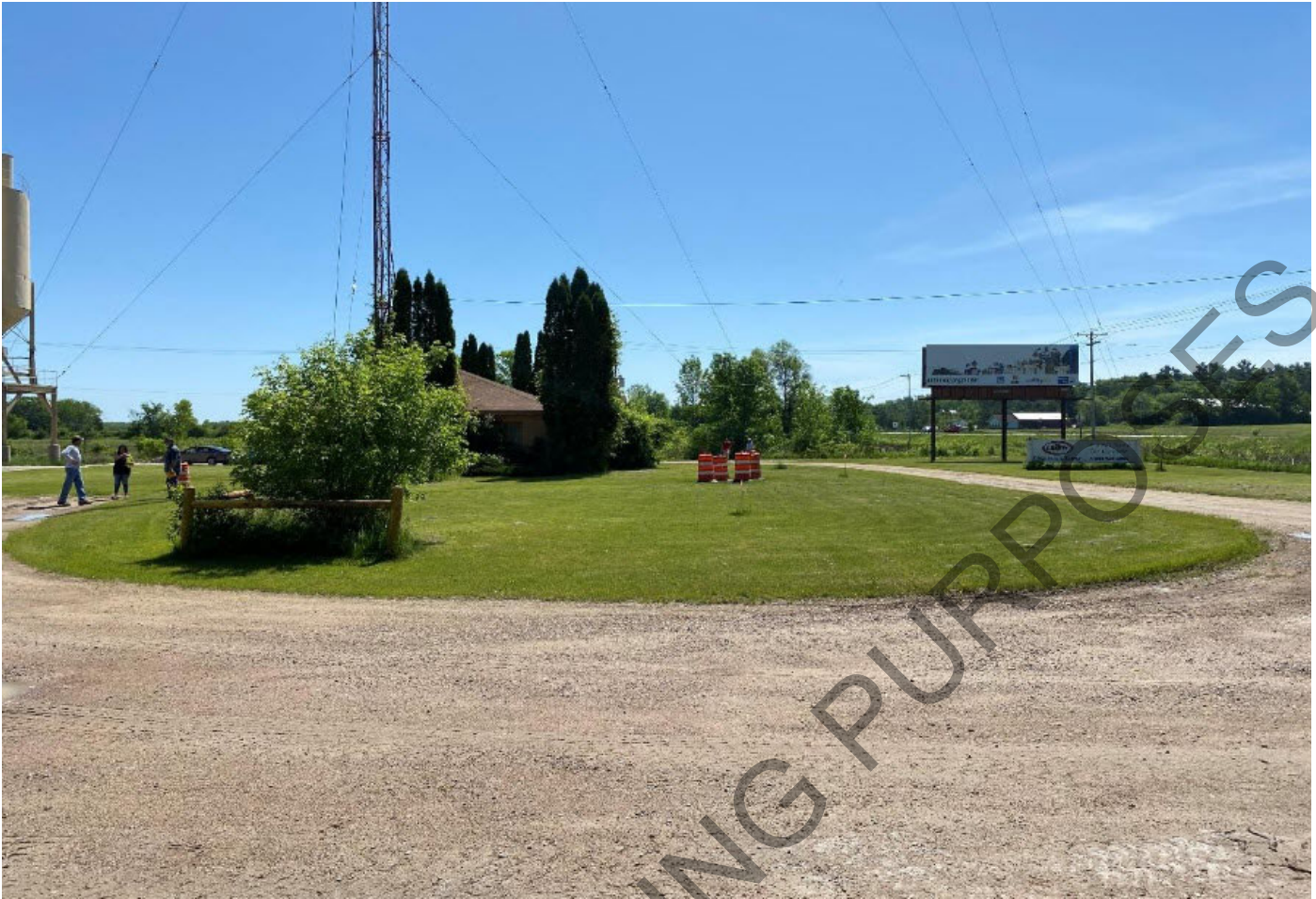
View of Tower, Sign, and Billboard
