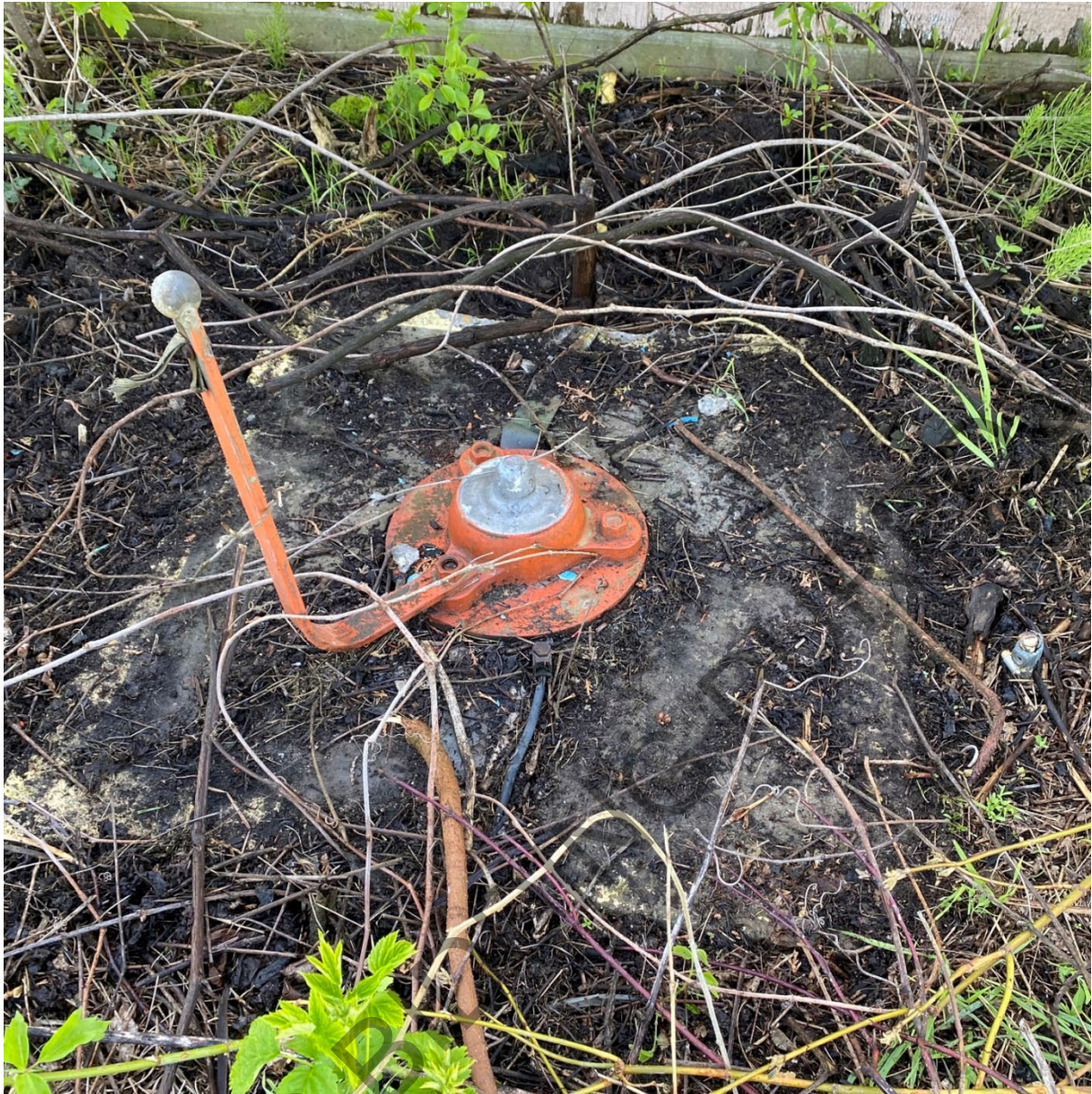
Tower Base (approximately 3' wide x 3' long)
