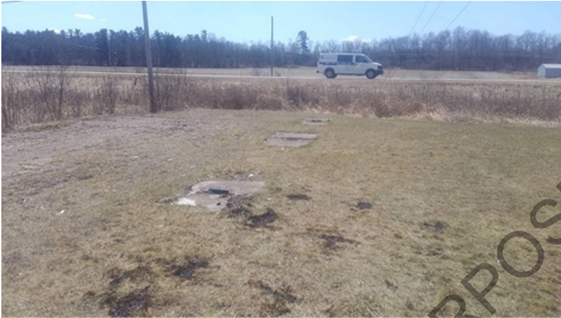
Three Concrete Footings From Billboard
