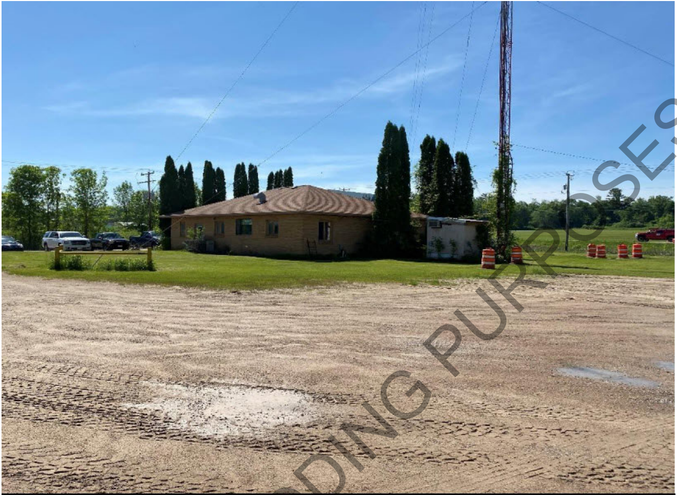
Tower and Guy Wires
