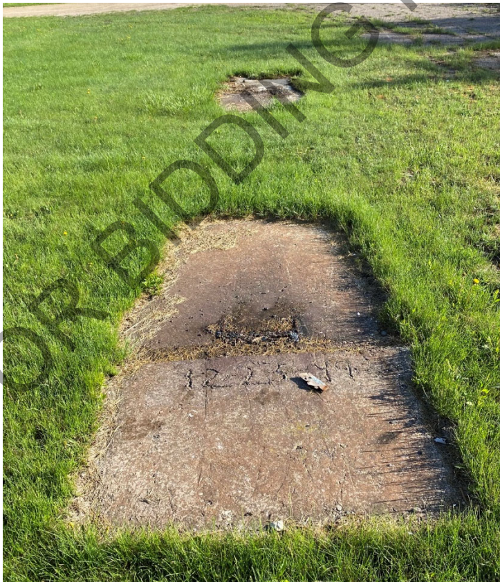
Concrete Footings From Billboard (approximately 8' long x 4' wide x 3' deep)
