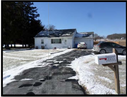
View from Hwy USH 51 facing west
